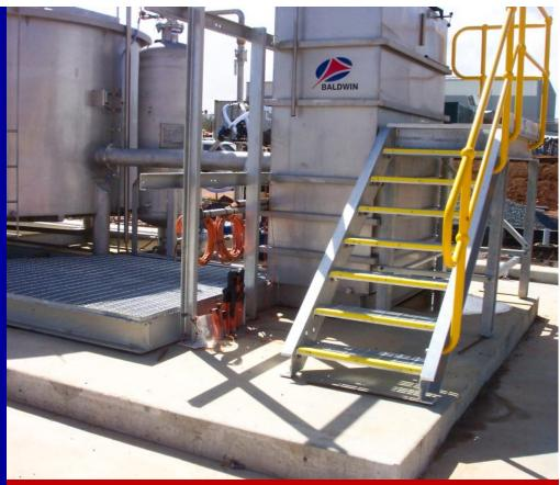
40,000L/Hr PLC Controlled Mine Site DAF
