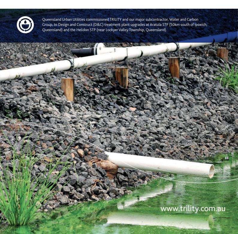
The Design and Construction (D&C) of the free water surface wetlands at the Aratula and Helidon Sewage Treatment Plants (STPs) will ensure licence compliance (Biochemical Oxygen Demand/Suspended Solids (BOD/SS)) ahead of projected flows at each site of between 80kL/day-200kL/day and 220kL/day, respectively. Feasibility studies at both sites found that constructed wetlands would ensure licence compliance in the long term and produce significantly lower effluent in the short term.
