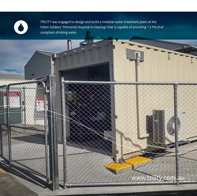
TRILITY designed, built, installed and commissioned a bespoke, modular water treatment plant to ensure the bore water supply at the Fallen Soldiers' Memorial Hospital complied with the Drinking Water Standards for New 7ealand.
