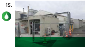
Hawke's Bay District Health Board Main Water Supply and Treatment System TRILITY was engaged to design, build, install and commission a bespoke modular water treatment plant at the Fallen Soldiers' Memorial Hospital in Hastings that is capable of providing 1.3 ML/d of compliant drinking water.
