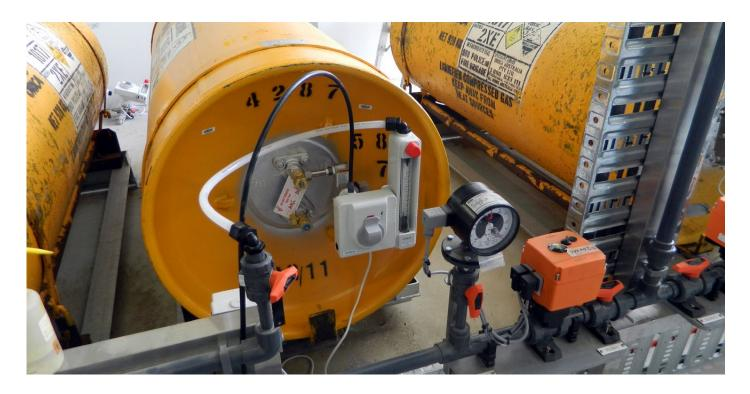
The TRILITY regulator exchange programme swaps over existing Wallace and Tiernan vacuum regulators with refurbished ones. Changing the PM kit onsite is not a full service. When TRILITY removes the regulators from site they are overhauled and refurbished in a workshop environment.
